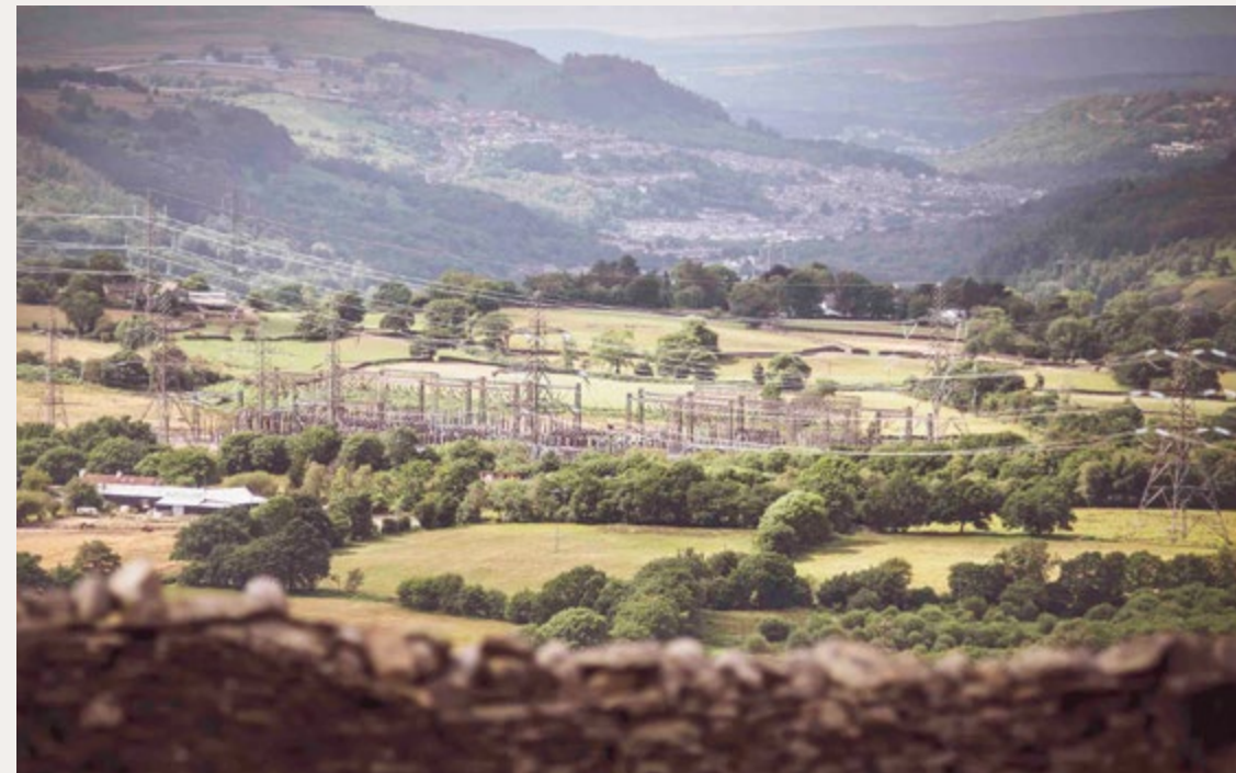
Upgrading Grid Capacity to Accommodate Renewable Generation
